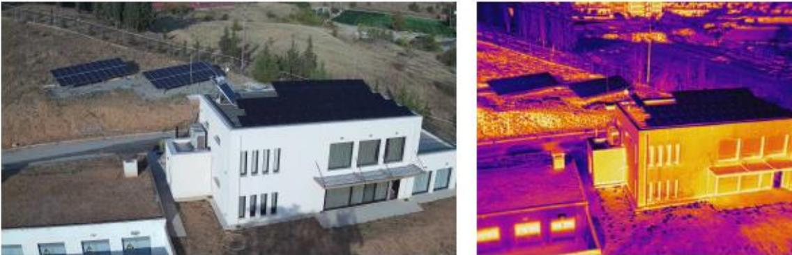
Fig. 4: Example input pair. An optical camera frame (left) and corresponding thermal input frame (right). Images were captured with cameras mounted on an Unmanned Aerial Vehicle (UAV), surveying the structure of interest.
