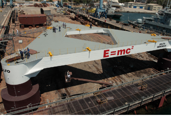
Fig. 1. The triangular marine platform during construction. Source: http://www.inp.demokritos.gr/nesor/dberenike/index.html .
